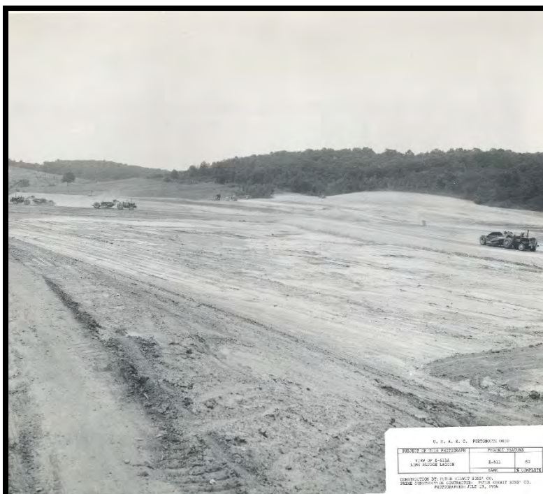
Figure 12: Excavation Work for the X-611A Lime Sludge Lagoon, July 1954
